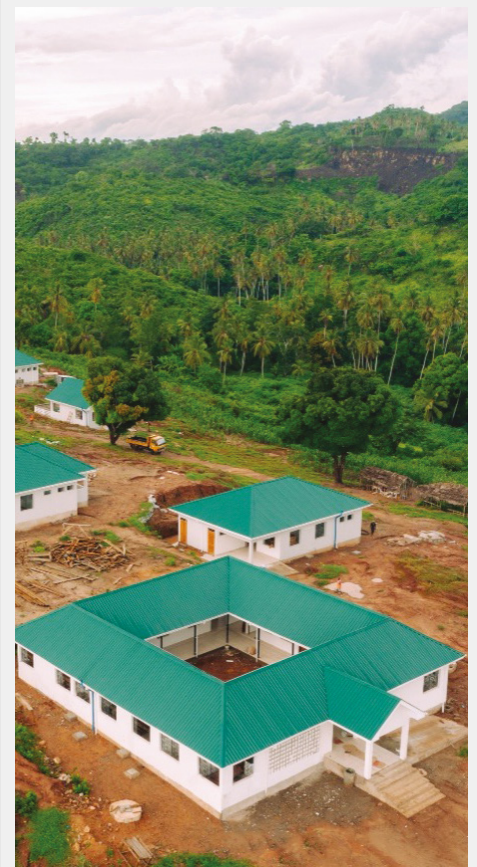
Construction in progress at Chumo Health Center
