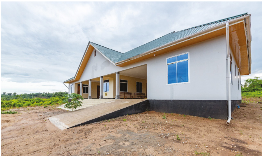
Dispensary Building at Nahama Village
