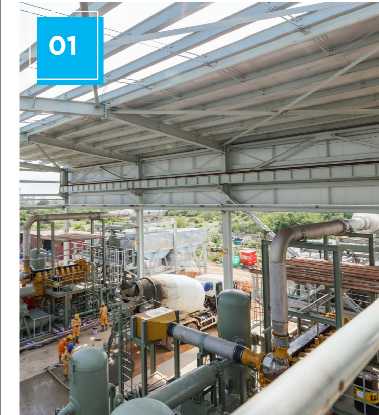
Strengthen the availability and reliability of electrical power by increasing generation capacity, transmission, and distribution networks.
