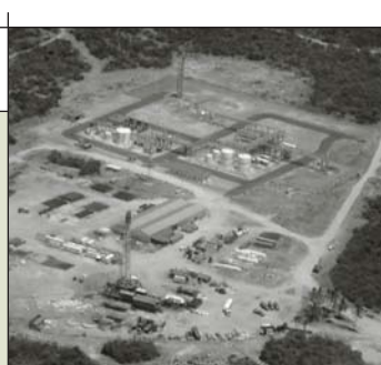
RIGHT AND OPPOSITE PAGE The new SS-10 well was drilled adjacent to the Songo Songo gas processing plant.
