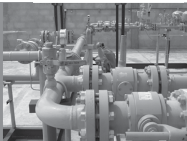
FAR LEFT: The new Wazo Hill cement plant kiln #4 is operating on Additional Gas supplied by Orca.
